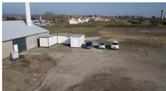
Centre Technique Municipal
